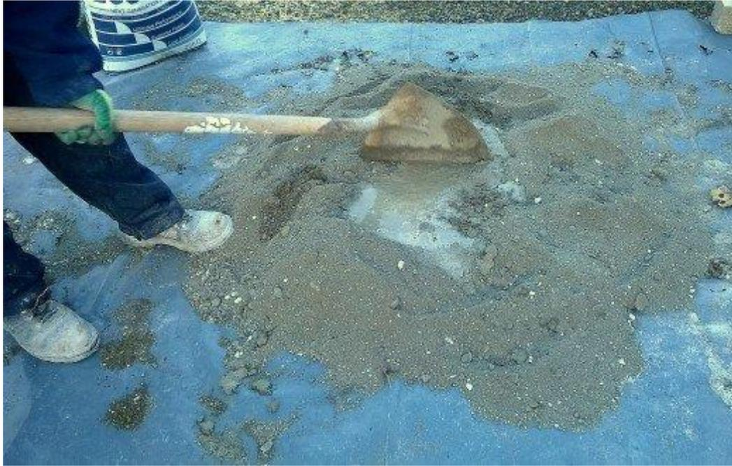
*“Chop” the pile with the edge of the shovel to help distribute the water. Continue to add water | Source*
