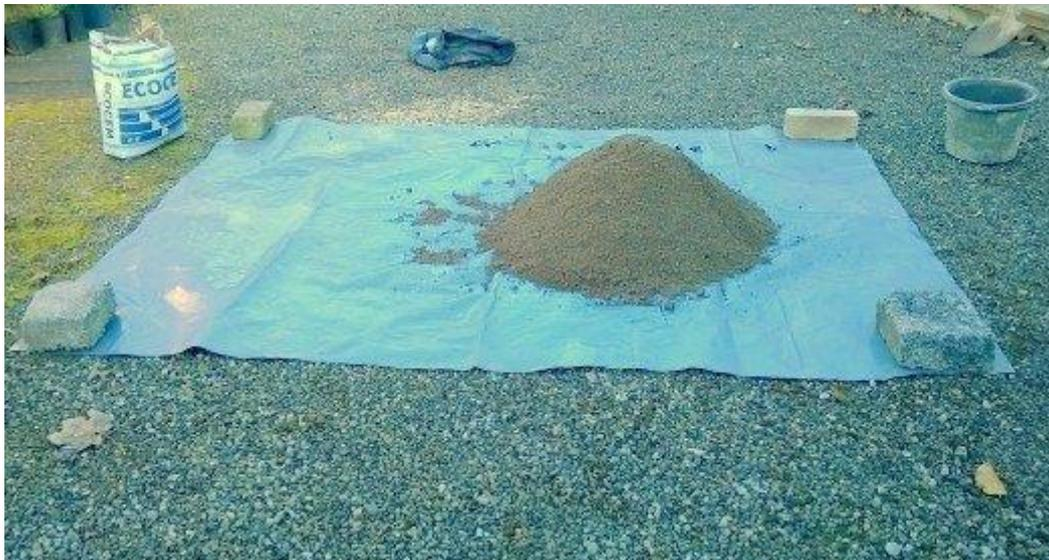
*Measure out the stone first and tip the sand on top. Keep the pile to one side of centre so you can mix sideways | Source*
