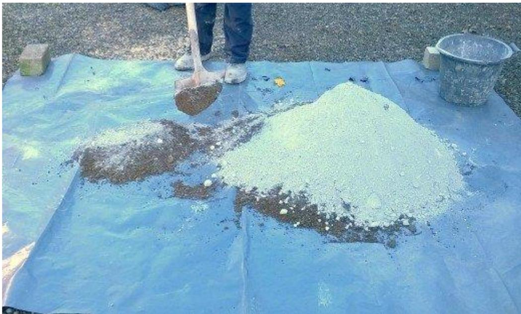
*Shovel the pile to one side, taking the material from the bottom edge. Do this 4 times in total*
