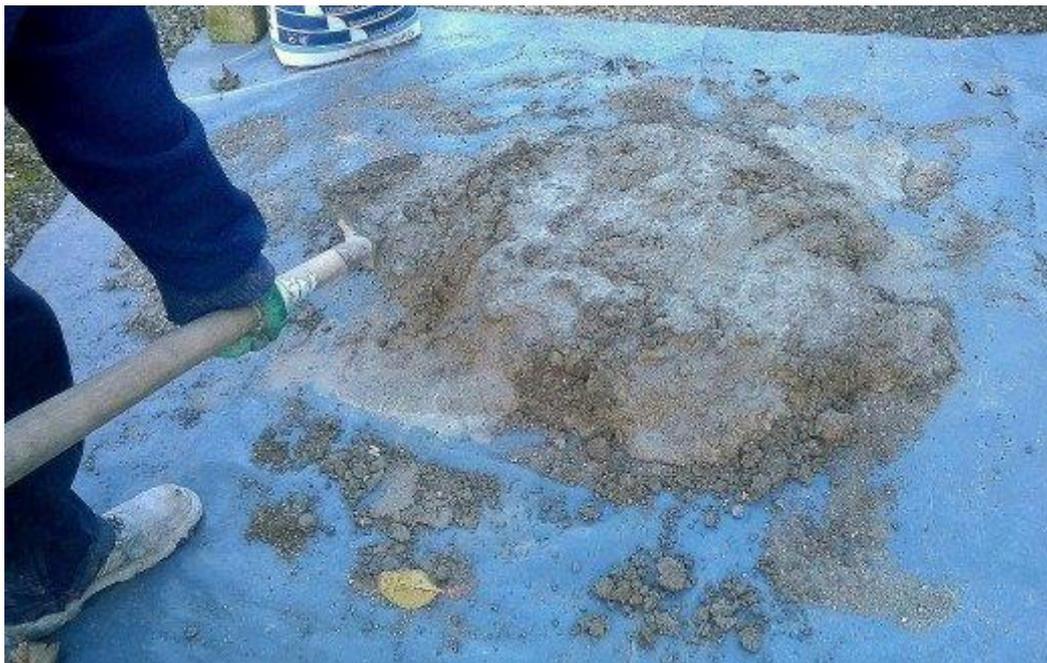
*Continue to add water as needed and walk around the perimeter of the pile, folding the mixture towards the centre and “chopping” | Source*
