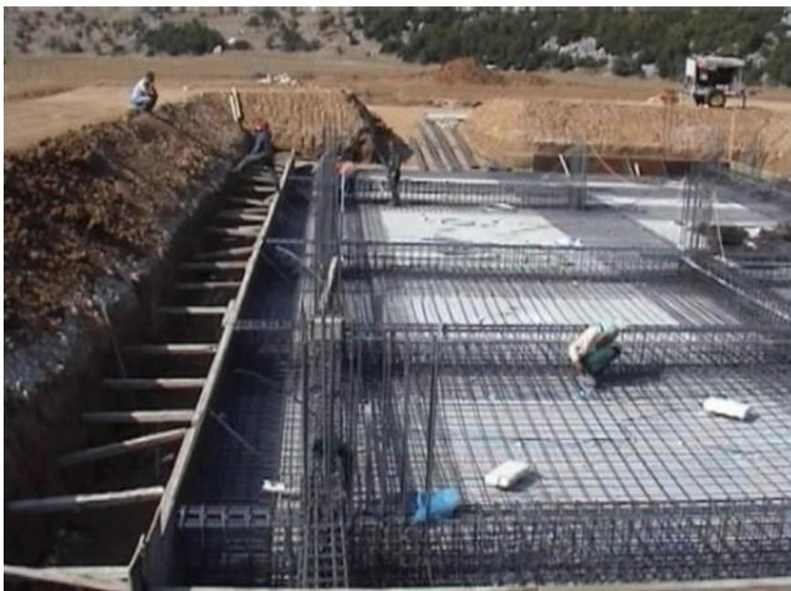
This type of foundation is useful for public buildings, office buildings, school buildings, residential quarters etc., where the ground conditions are very poor and bearing power of the soil is so low that individual spread footing cannot be provided.
